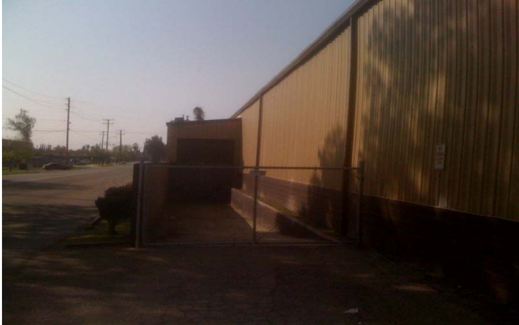
Recessed loading dock w/dock leveler
